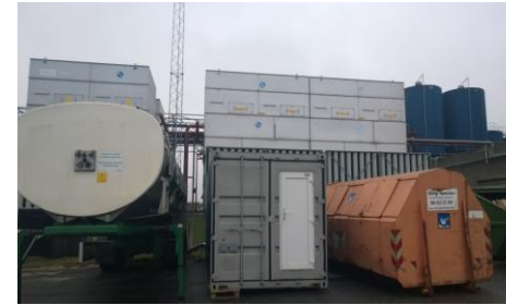
Cooling tower re-use
